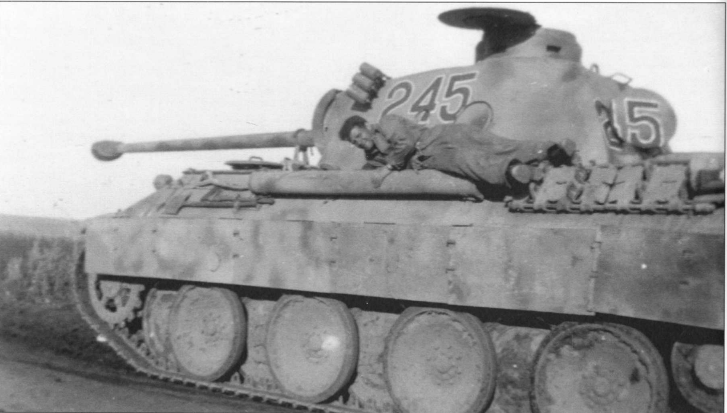
A Panther halted on a road. One of the crew poses for the camera sprawled out across the vehicle's cleaning tube. The Panther still retains its old smoke candle dischargers that were fitted on either side of the turret. This practice ceased in June 1943 after a reported incident earlier that year, when enemy small arms had set off the dischargers, incapacitating the crew.
