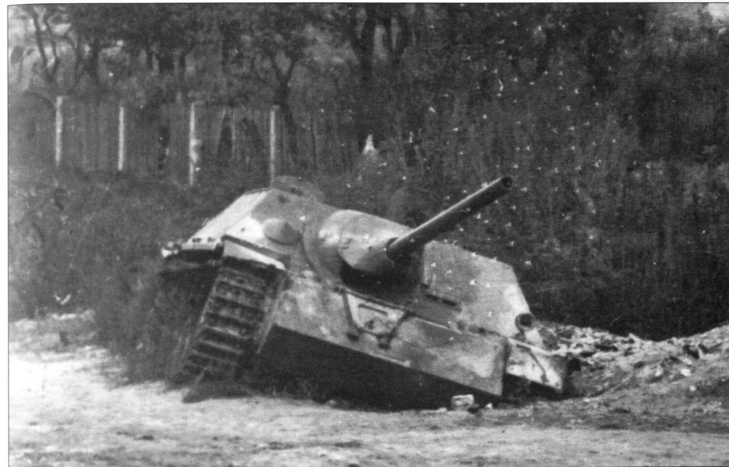
Three photographs showing abandoned Jagdpanzer IV's. With a drastic need for new armoured fighting vehicles, more second generation tank destroyers were built. One such vehicle that came off the production line in 1944 was the Jagdpanzer IV. This vehicle, built on the chassis of a PzKpfw IV, weighed 28.5 tons and was nicknamed 'Guderian's duck'. The vehicle was equal to any enemy tanks thanks to its potent 7.5cm gun. The Jagdpanzer saw extensive service in the east and with its reliability and well-sloped thick frontal armour it became a highly efficient fighting vehicle, if only for a short period of time.
