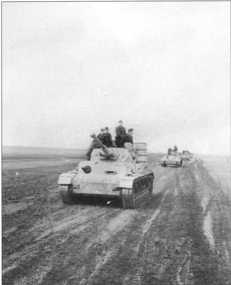
A column of PzKpfw IV's move along a typical road in southern Russia during operations in the early winter of 1943. Stowed on the rear of the engine deck of the leading vehicle are fuel drums. The vast distances in which these vehicles were compelled to travel meant that quite often tracked vehicles outstripped fuel supplies, prompting crews to carry reserves.
