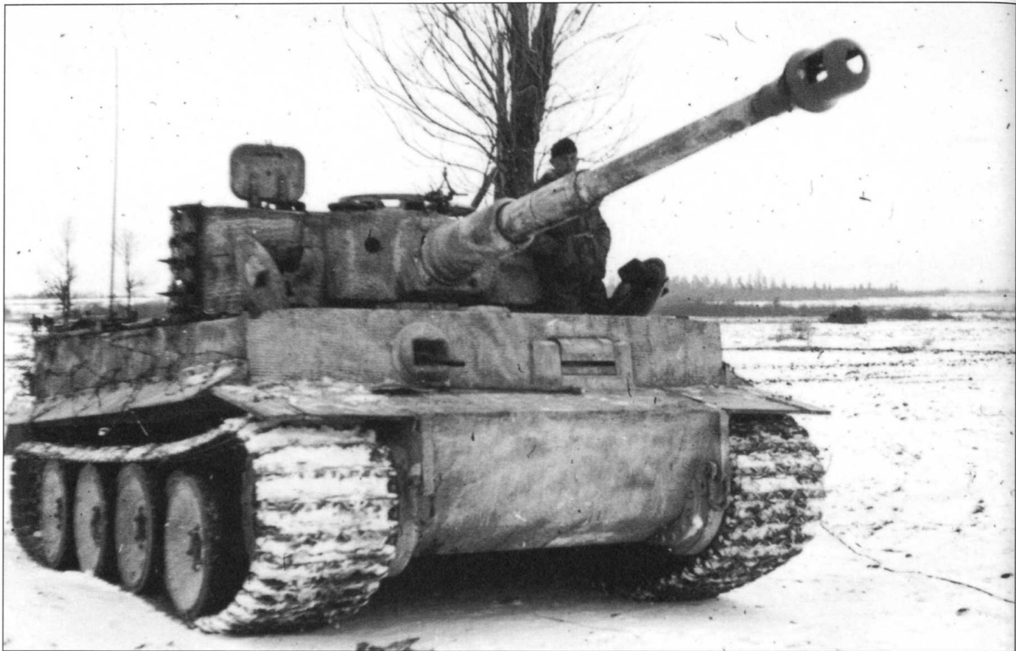
Two photographs showing Tiger tanks with an application of winter whitewash paint over a coating of Zimmerit anti-magnetic mine paste. By early 1944 the Tiger continued to play an important, mainly defensive, role.
