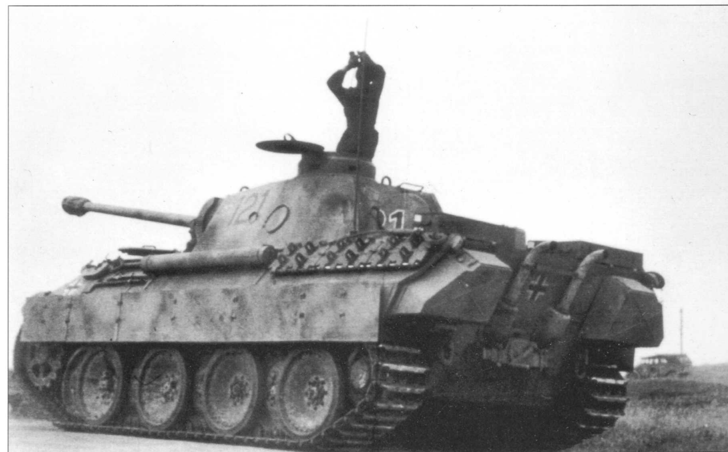
Two photographs showing the same Panther Ausf G during operations on the Eastern Front in autumn 1944. The improved Ausf G had improved new vision devices and thicker side armour. Some of them had all-steel road wheels and a number had an early infrared sighting device – technology that was well ahead of its time.
