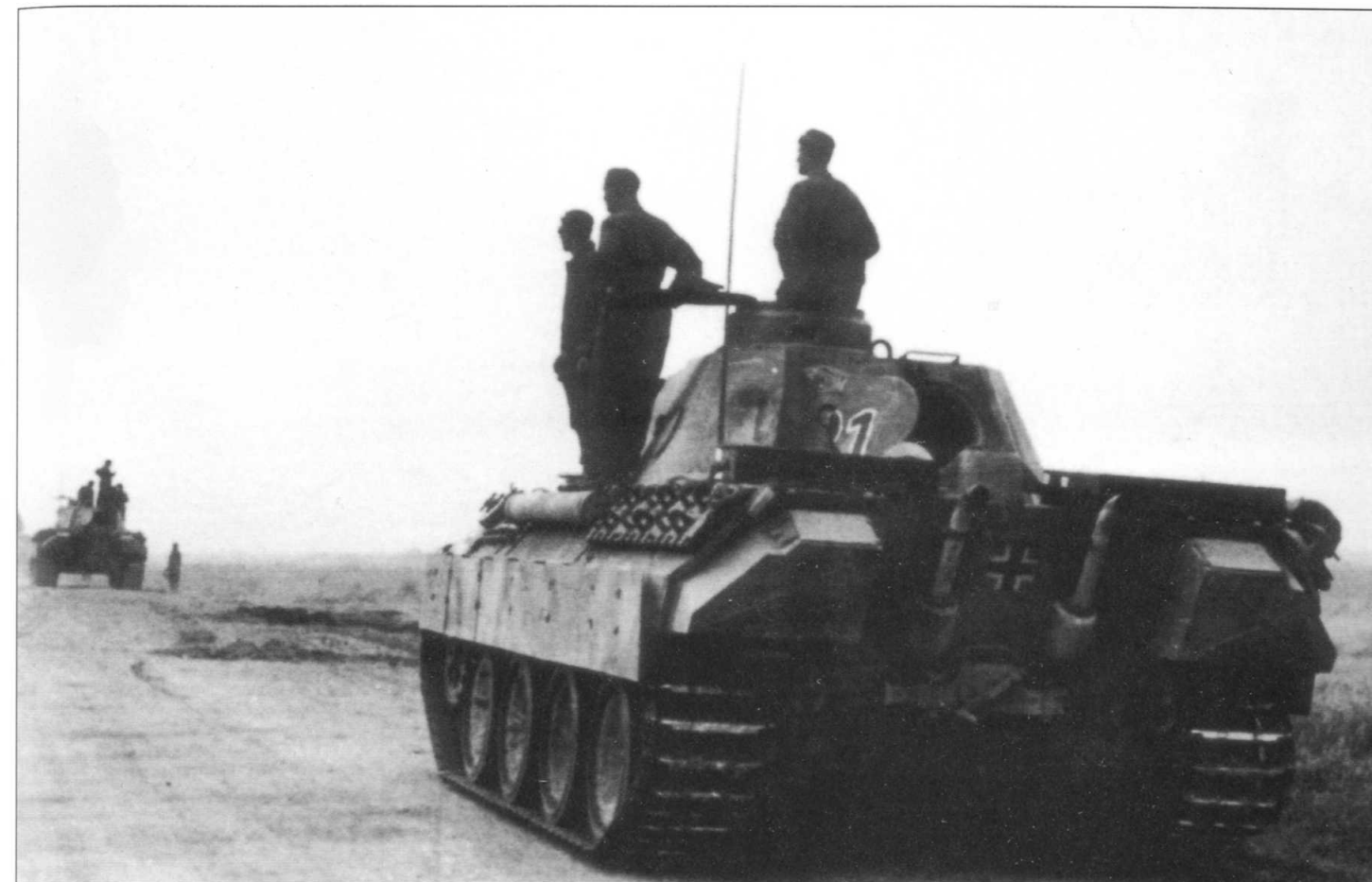
Two photographs showing the same Panther Ausf G during operations on the Eastern Front in autumn 1944. The improved Ausf G had improved new vision devices and thicker side armour. Some of them had all-steel road wheels and a number had an early infrared sighting device – technology that was well ahead of its time.
