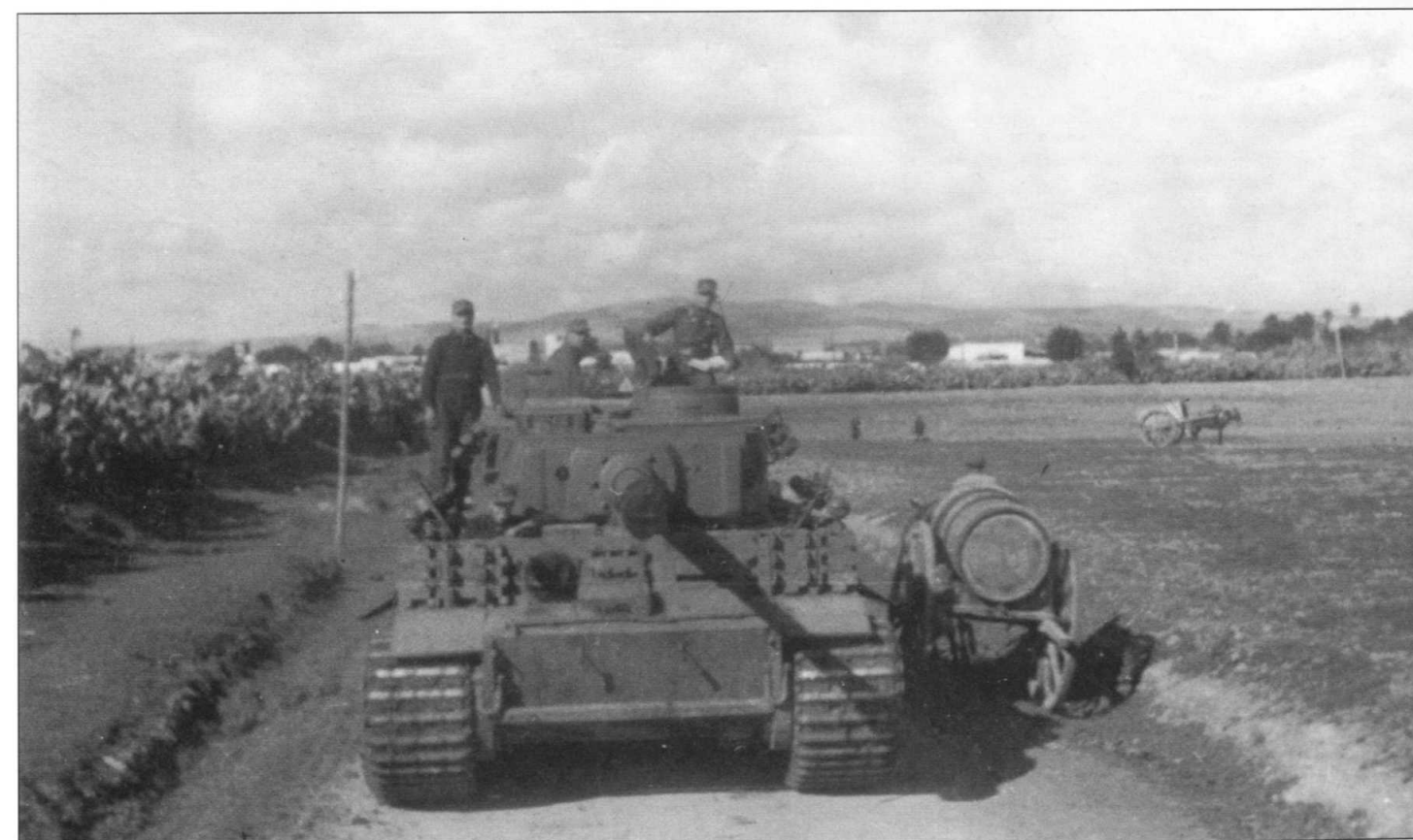
A Tiger rumbles along a road during the autumn of 1944. Track links have been bolted to the front of the tank for additional armoured protection.
